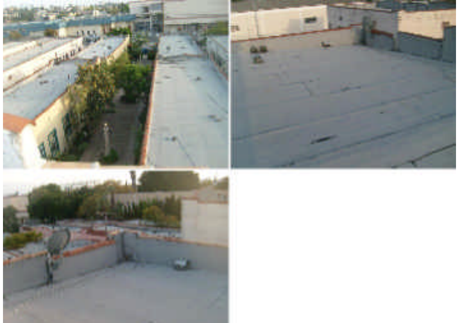
Upper roof & looking down on lower roofs
