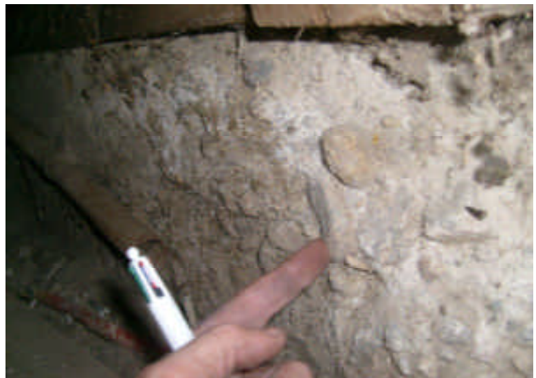
Older foundation with round aggregate
