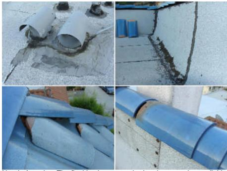
Needs Attention: The flashing is not standard and may not be a reliable installation, it will require high maintenance to ensure that it remains leak free. The mastic is cracked in areas and is not reliable to ensure a watertight seal.
