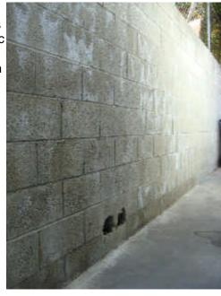
There is accumulated debris between the walls along the right side, and the neighboring wall appears to be leaning out of plumb. This area does not appear to have proper drainage.
