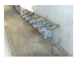
CONDITION: There is no automatic seismic gas shut-off valve on the main gas line.
