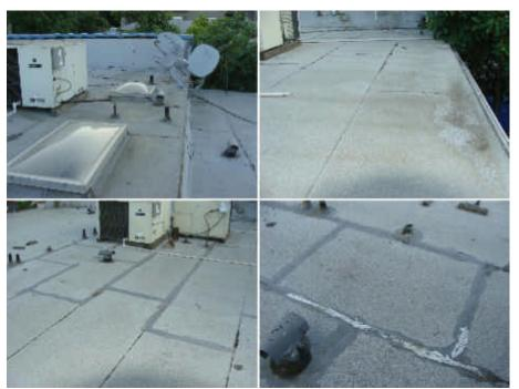
Needs Attention: On the low sloped / flat roof, there are bubbled areas of roofing material and the roof deck is soft under foot. This is an indication that some moisture has gotten under the material.
