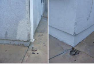
are deteriorated at the right front and right rear corners of the building (It appears the protective pipes have been removed and there has been contact from autos.).
