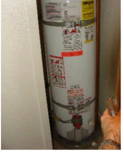
Not Acceptable: This does not have the necessary openings/ grills to allow the required fresh air for combustion.
